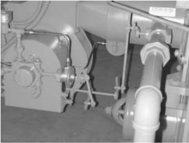
Figure 6-1: Complete Linkage Assembly - Combination Gas and Oil
