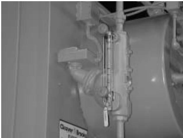
Figure 1-4: Low Water Cut Off (LWCO)
