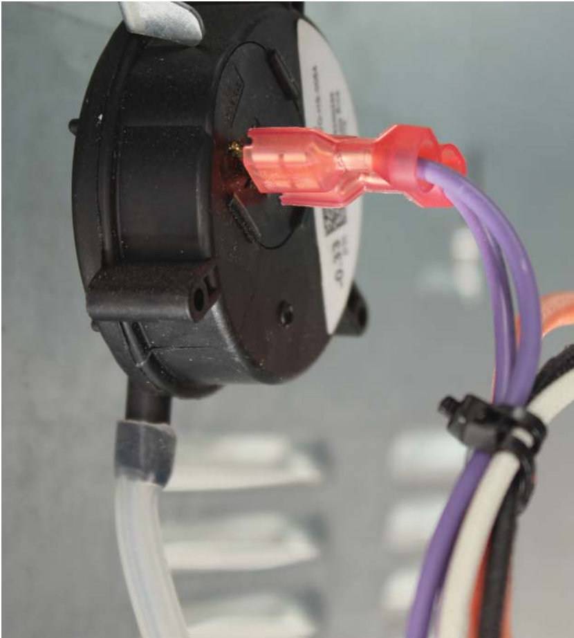
Figure 5 - 2 Combustion air pressure switch
