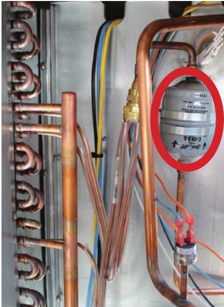
Figure 3 -4 Filter-drier
