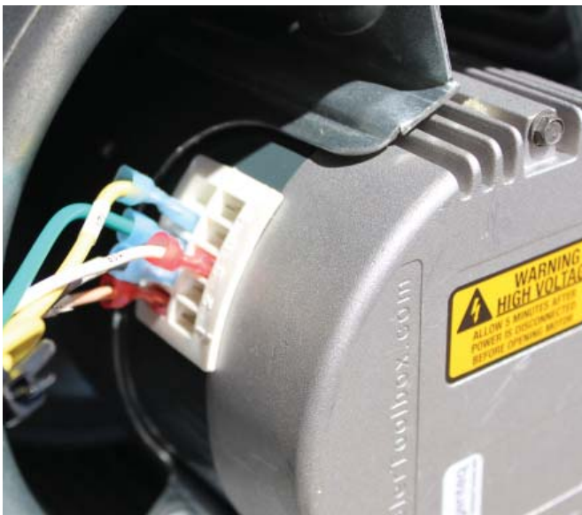
Figure 3 -8 X-13 blower motor
