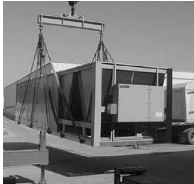
FIG. 2 – UNIT RIGGING
