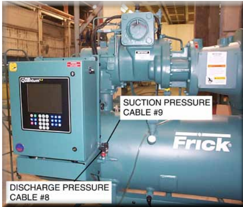
Figure 27a. Wiring Harness Installation, RXF 58 – 101.
