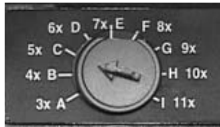
Figure 18: Circuit Breaker Trip Adjustment Dial
