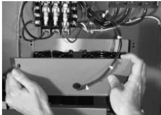
Figure 31: Remove the Heatsink Fan Assembly
