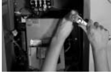
Figure 25: Remove Picture Frame Screws
