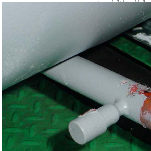
Figure 35 - High Flow Shradder with Cap
