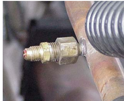
Figure 4. Fuse/Fusible Plug Relief Device and Fitting (should never be capped)
