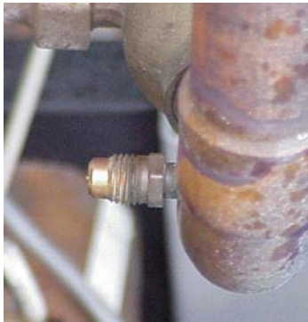
Figure 3. Standard Schrader Access Valve and Fitting
