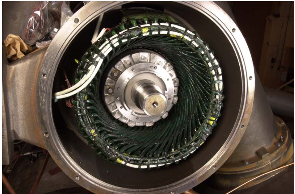
Figure 1: CVHF 1470 or 1720 with thrust bearings removed. The bearing cap seal is shown in place in preparation for a new thrust bearing installation. Note: A gasket is not used on the bearing cap.
