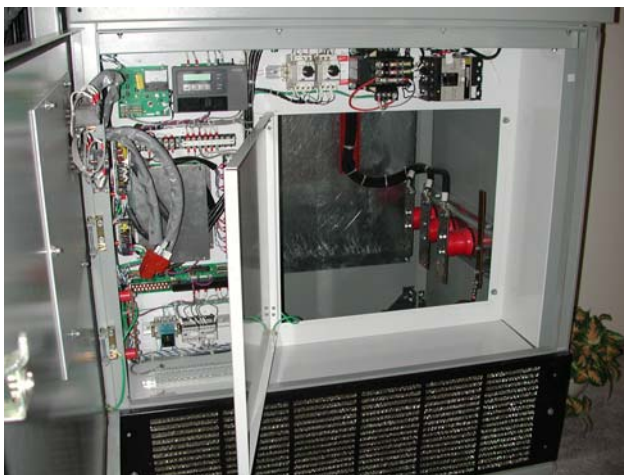
Fig. 10 – Access door to motor lead connection bus
