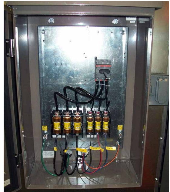
FIGURE 99 - SINGLE POINT POWER CONNECTION
