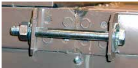
Raceway Lifting Lugs Assembled
