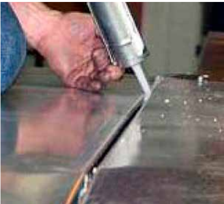
FIGURE 50 - APPLYING CAULK TO SEAMS
