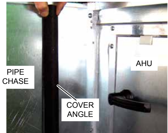
FIGURE 92 - INSTALL COVER ANGLE
