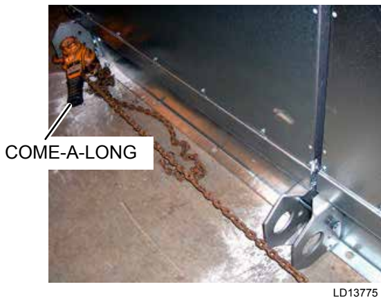
FIGURE 56 - COME-A-LONG ATTACHED TO A SECTION
