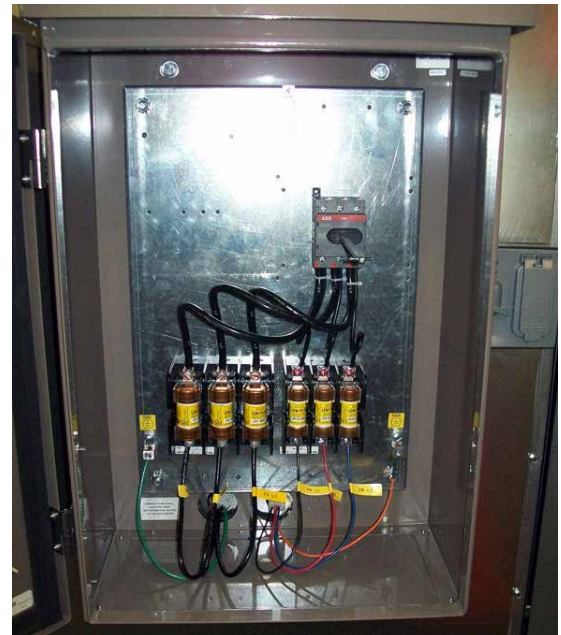
FIGURE 39 - SINGLE POINT POWER CONNECTION
