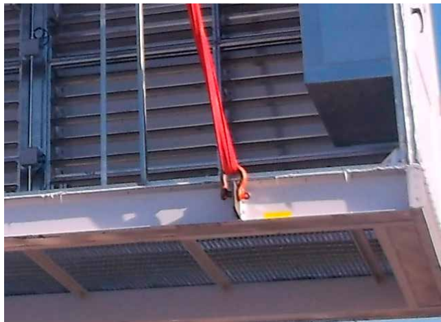
FIGURE 6 - PROPER LIFTING WITH BASE RAIL
