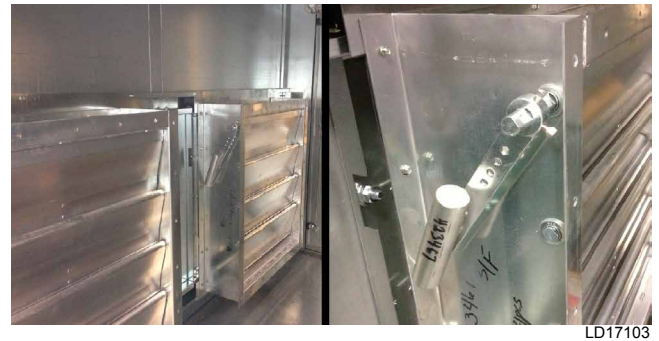
FIGURE 26 - COUNTERBALANCE LOCKED INTO PLACE FOR SHIPPING
