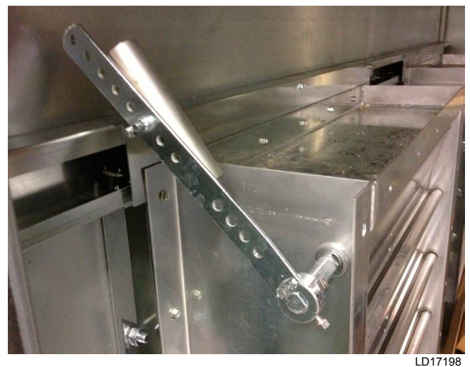
FIGURE 27 - COUNTERBALANCE UNLOCKED FOR START-UP
