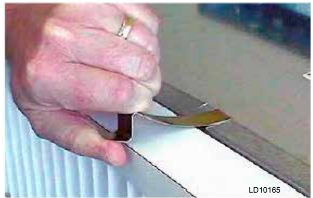
FIGURE 100 - POSITION PRE-FILTER IN FRONT OF FINAL FILTER
