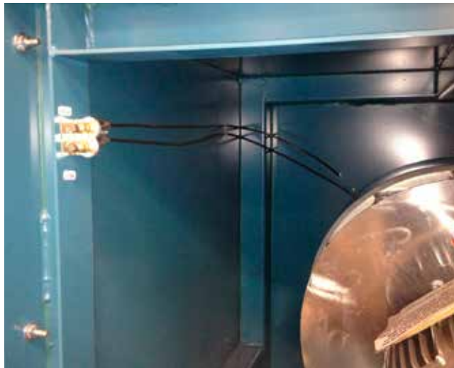
FIGURE 11 - HIGH AND LOW CONNECTIONS AND ASSOCIATED TUBING FOR FAN MOUNTED AIR MONITORING SYSTEM
