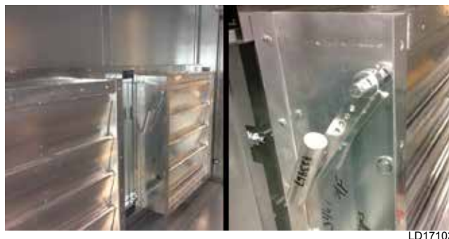
FIGURE 5 - COUNTERBALANCE LOCKED INTO PLACE FOR SHIPPING
