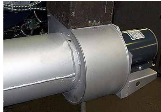
FIGURE 32 - FLUE COMBUSTION TEMPERATURE AND EFFICIENCY TEST PORT- ID BLOWER
