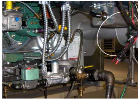
FIGURE 30 - CHECK MAIN GAS SUPPLY PRESSURE
