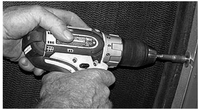
FIGURE 73 - LOOSEN SCREWS BEFORE ADJUSTING SEALS
