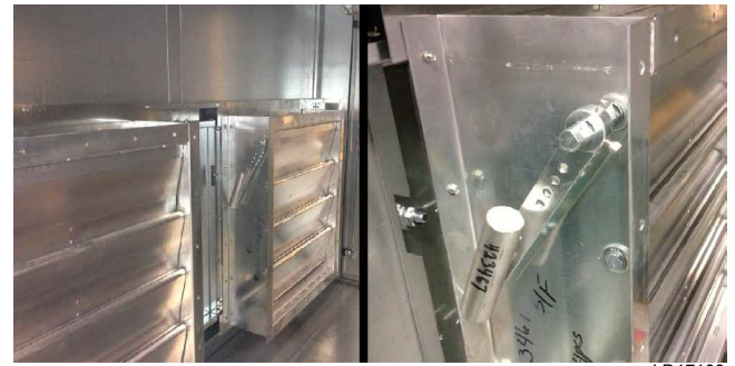
FIGURE 6 - COUNTERBALANCE LOCKED INTO PLACE FOR SHIPPING
