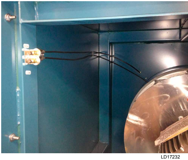
FIGURE 12 - HIGH AND LOW CONNECTIONS AND ASSOCIATED TUBING FOR FAN MOUNTED AIR MONITORING SYSTEM
