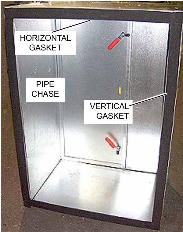
FIGURE 86 - APPLY GASKET TO PIPE CHASE
