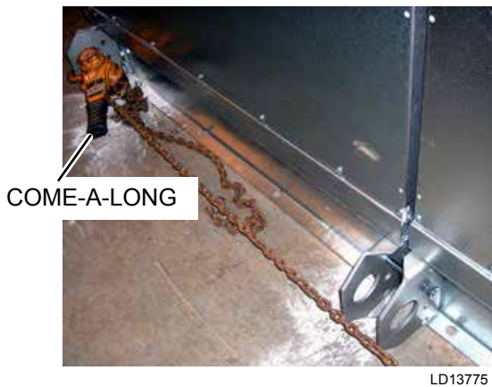
FIGURE 56 - COME-A-LONG ATTACHED TO A SECTION
