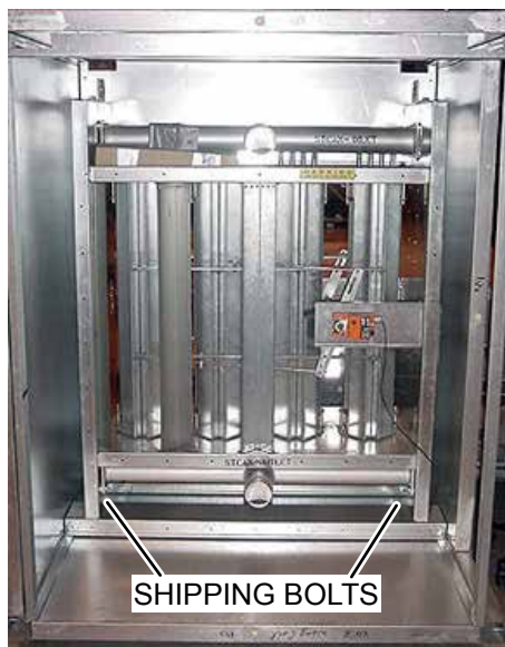
FIGURE 123 - VIFB COIL (FACE-MOUNTED ACTUATOR SHOWN)
