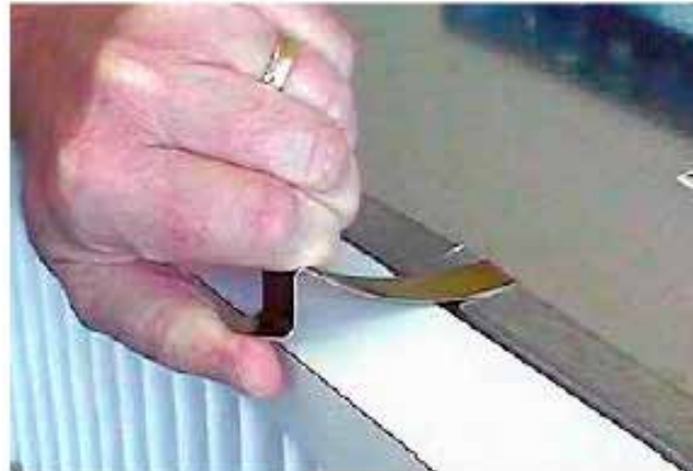
FIGURE 162 - POSITION PRE-FILTER IN FRONT OF FINAL FILTER
