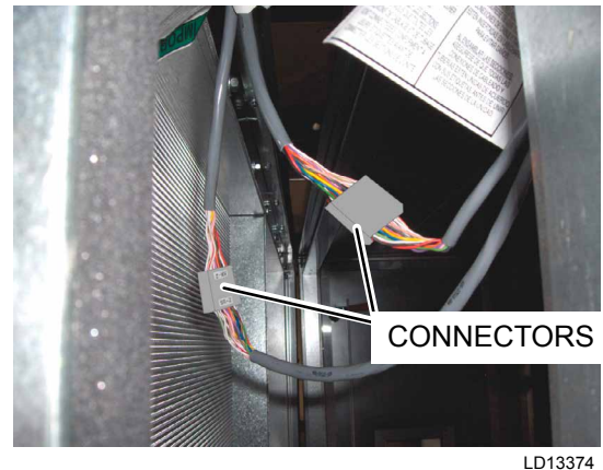
FIGURE 59 - ELECTRICAL CONNECTORS (CONNECTED)
