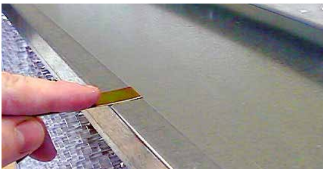
FIGURE 161 - INSTALLING PRE-FILTER LATCH
