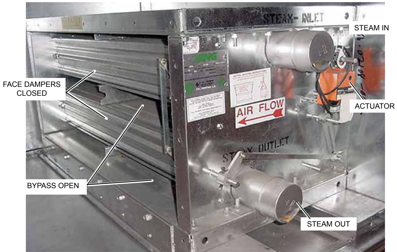
FIGURE 122 - IFB COIL (HORIZONTAL TUBES AVAILABLE WITH STEAM AND HOT WATER)
