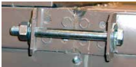
Raceway Lifting Lugs Assembled
