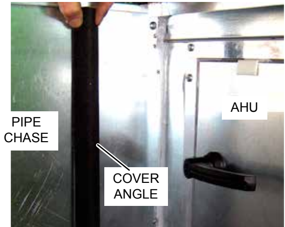
FIGURE 92 - INSTALL COVER ANGLE
