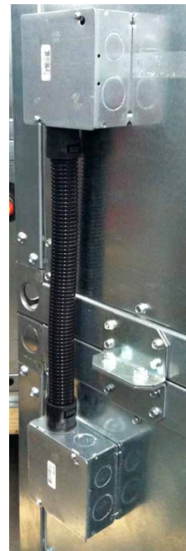
FIGURE 40 - CONDUIT (P/N 025-39024-001) AND SJO CORD (P/N 025-35746-001)
