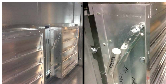
FIGURE 75 - COUNTERBALANCE LOCKED INTO PLACE FOR SHIPPING
