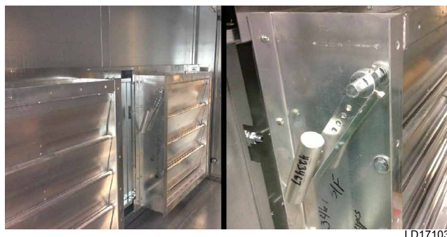
FIGURE 6 - COUNTERBALANCE LOCKED INTO PLACE FOR SHIPPING
