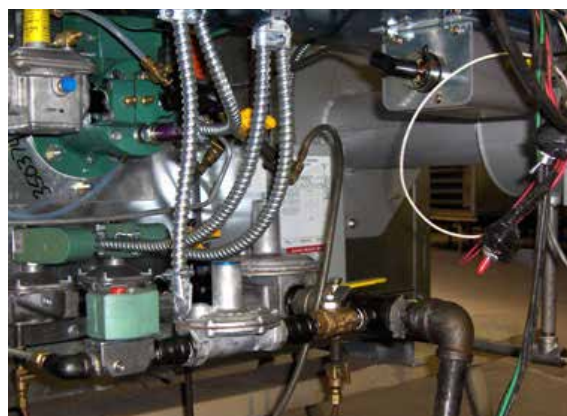
FIGURE 31 - CHECK MAIN GAS SUPPLY PRESSURE
