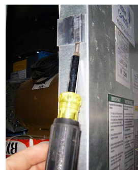
FIGURE 20 - METAL SPACERS ON SOLUTION XT DOORS
