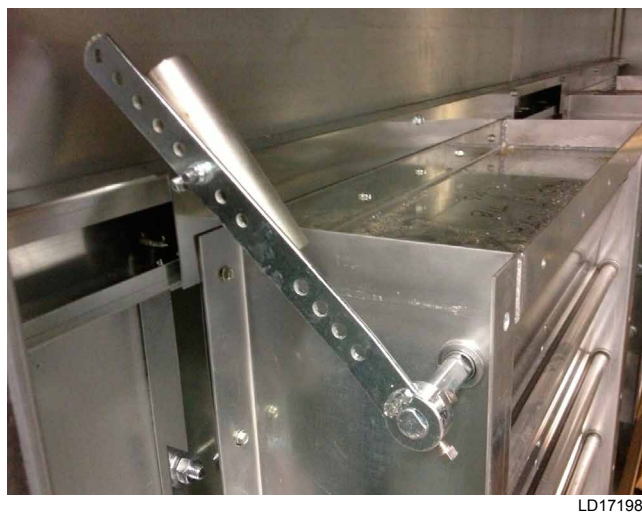
FIGURE 7 - COUNTERBALANCE UNLOCKED FOR START-UP
