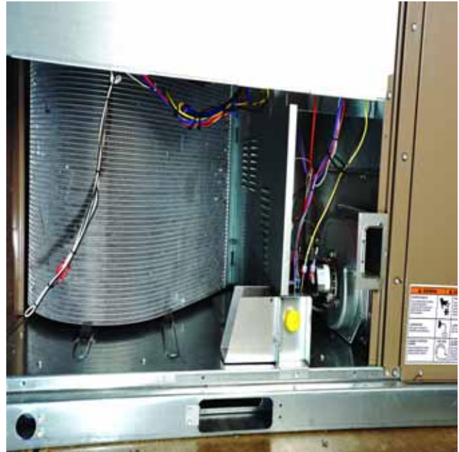
Figure 18: Flue Exhaust Hood Shipping Location
