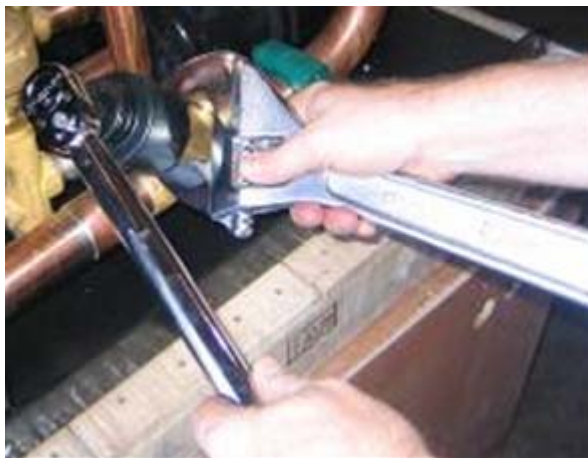
Figure 7: Valve and 41 mm Hex Socket
