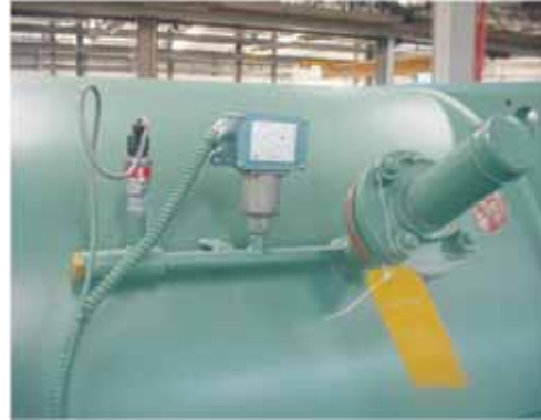
FIGURE 15 - RUPTURE DISK FROM FACTORY
