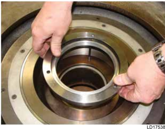
FIGURE 65 - EYE SEAL INSTALLATION
