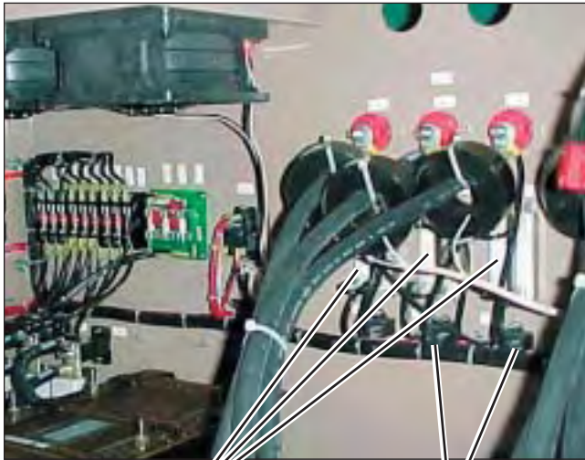
DV/DT RESISTORS
