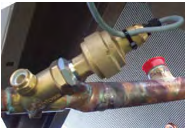
FIGURE 19 - ECONOMIZER STEPPER CONTROL VALVE
