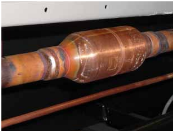
FIGURE 20 - CHECK VALVE
