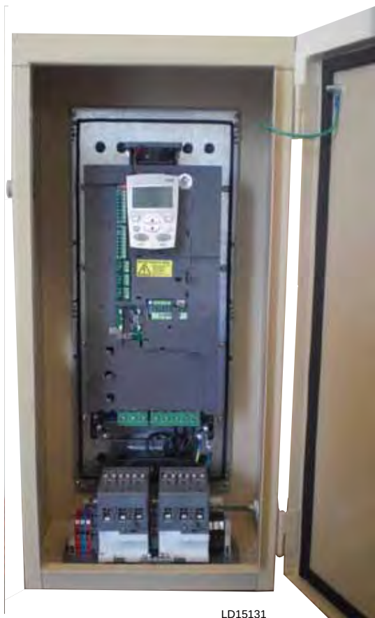
FIGURE 99 - INVERTER WITH KEYPAD AND DISPLAY INSTALLED
