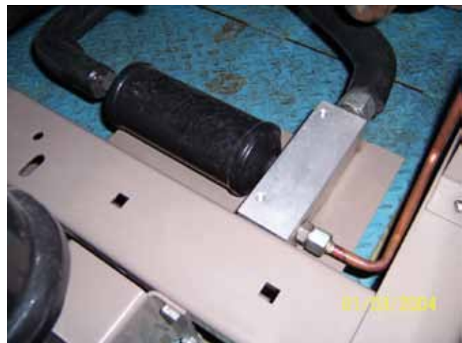
FIGURE 16 - EDUCTOR FILTER DRIER
