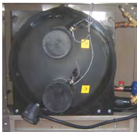
FIGURE 7 - 2-PASS EVAPORATOR WITH OPTIONAL IMMERSION HEATER
