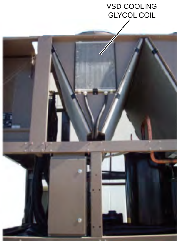
FIGURE 24 - GLYCOL COOLING COIL
