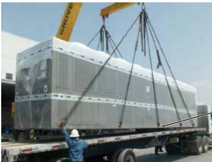
FIGURE 4 - PROPER LIFTING OF YVAA CHILLER
