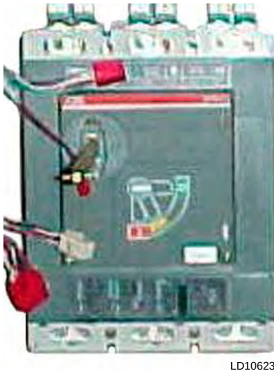
FIGURE 84 - CHILLER CIRCUIT BREAKER
