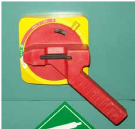
FIGURE 1 - EMERGENCY SHUTDOWN HANDLE
