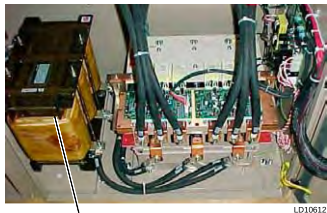
FIGURE 76 - 1L LINE INDUCTOR
