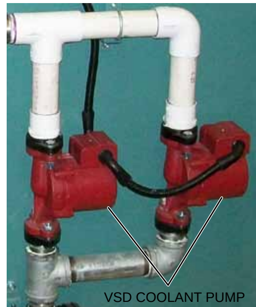
FIGURE 30 - VSD COOLANT PUMP
