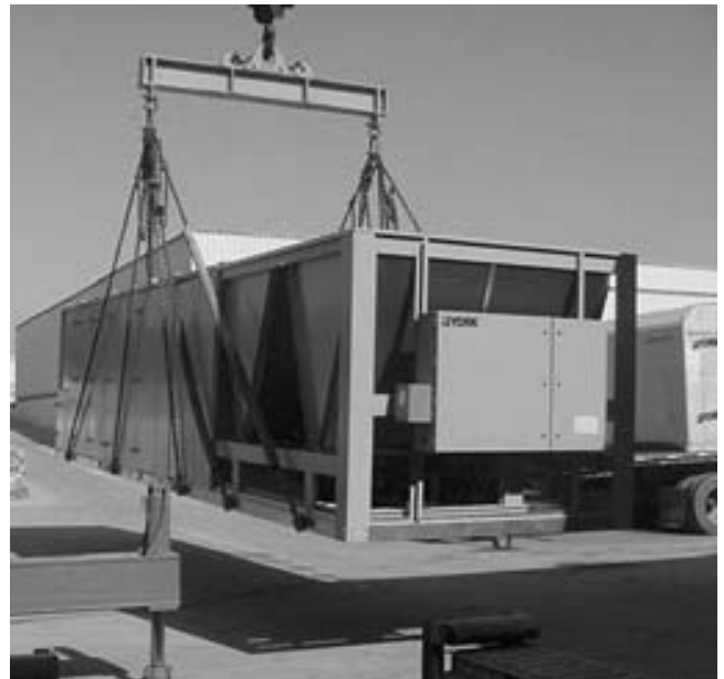
FIG. 2-2A – UNIT RIGGING
