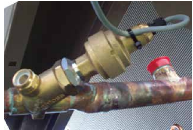
FIGURE 8 - ECONOMIZER STEPPER CONTROL VALVE
